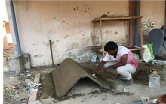
Fig 6: casting of specimen covered ferrocement
